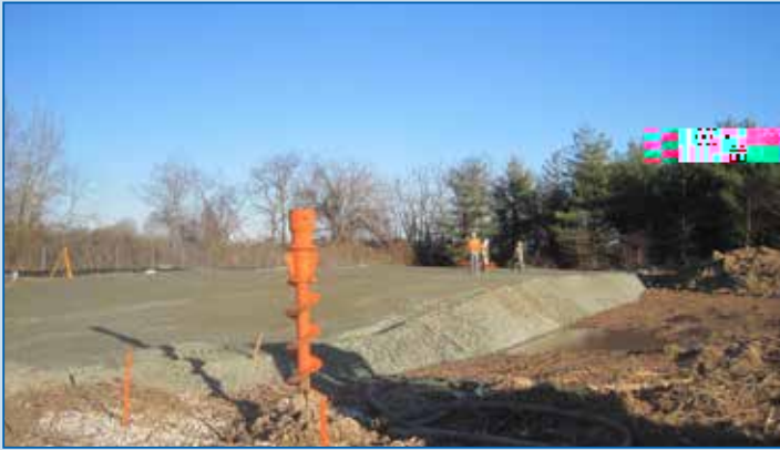
V jg"dwknfkipi"ukvg"ycu"i tcfgf"kp" Fgego dgt"cpf"Lcpwct {0" The treatment system building will measure 170 feet by 60 feet, by 36 feet high at the roof peak.
